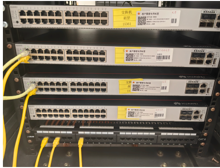
Figure 6: 机柜正面接线图
