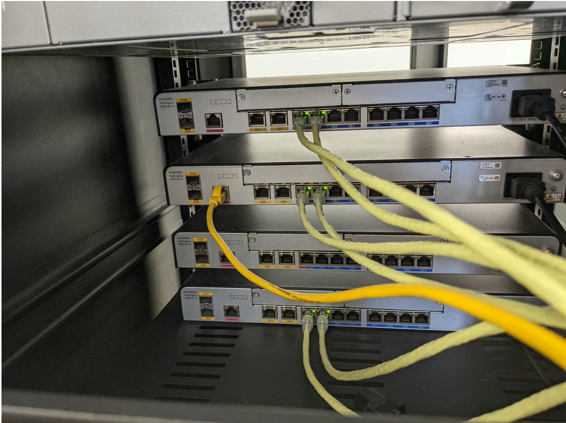
Figure 3: 机柜背面接线图
